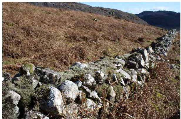
Fig. 6.9: Old dry-stone wall with Racomitrium lanuginosum . Feb. 2023.
