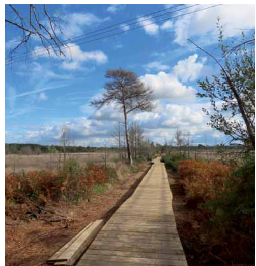
▽ Figure 2. Boardwalk replacement at Thursley, summer 2022.
